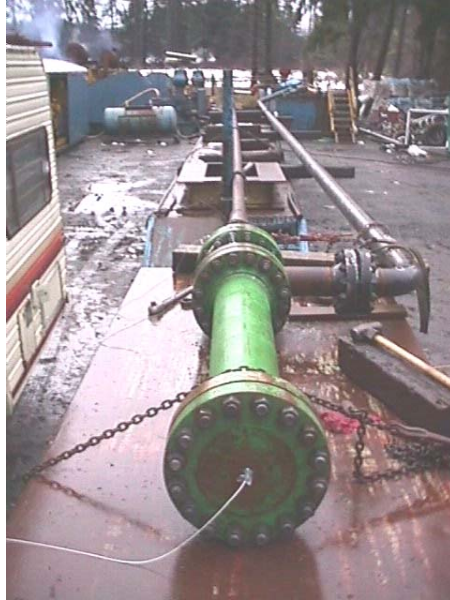
Figure 3. Flow loop test facility.
